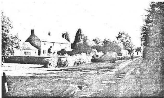
Former council houses
